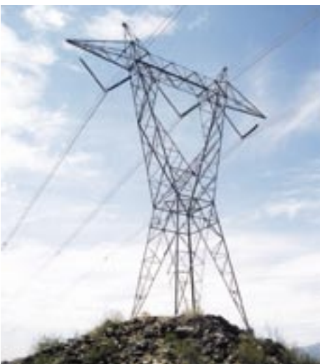
Transmission Line and Structure
