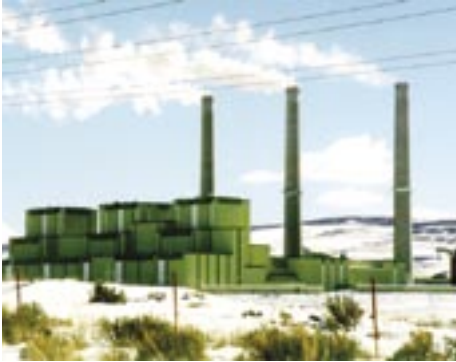
Steam-Electric Generation Plant
