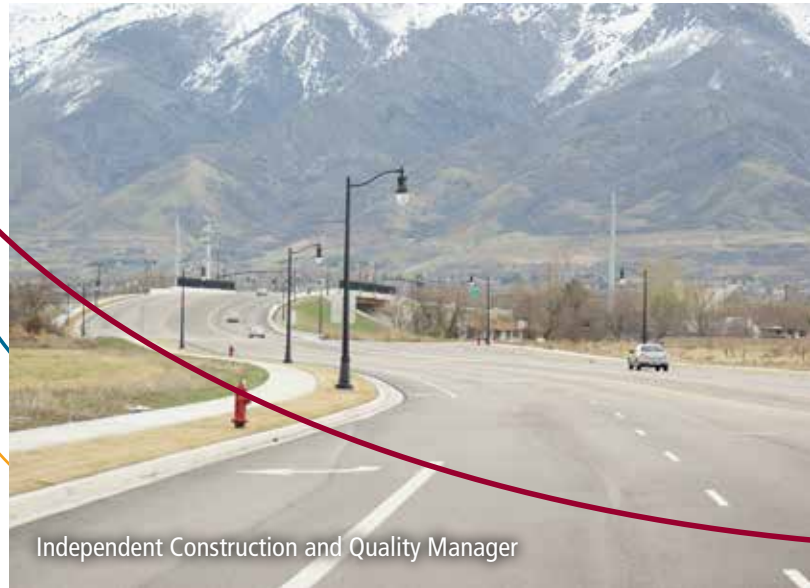
Accelerated Bridge Construction Owner's Engineer
