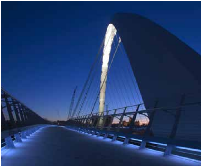
Pedestrian Bridge Construction Administration
