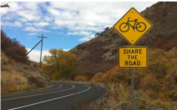
Bicycle Lane Road Widening
