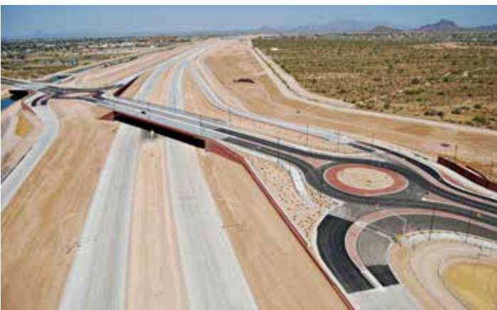
Diamond Interchange Using Roundabouts
