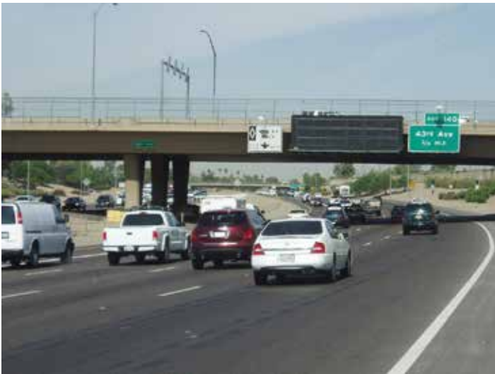
Freeway Signing and Pavement Marking
