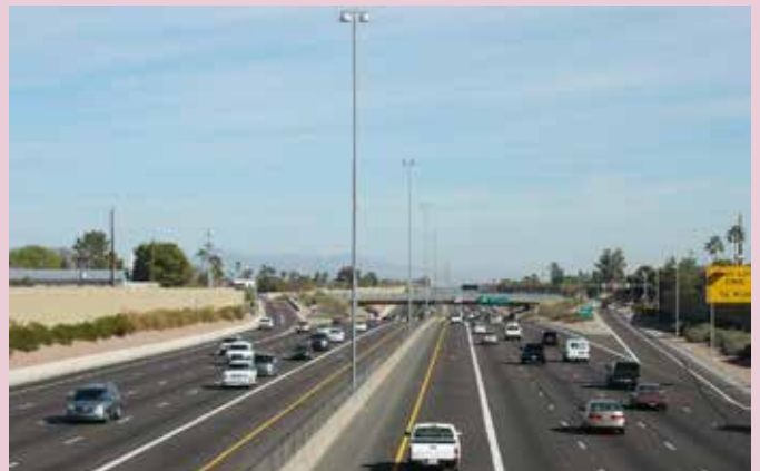
Overhead Lighting for Freeway
