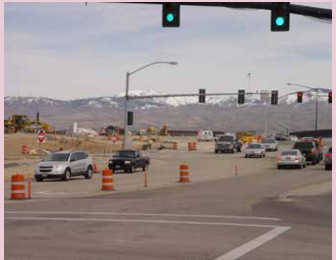
Maintenance of Traffic
